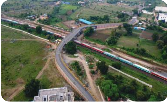
2 lane ROB at Railway Crossing (LC) – 293 between Bharatwada and Godhani Railway Stations in Nagpur
