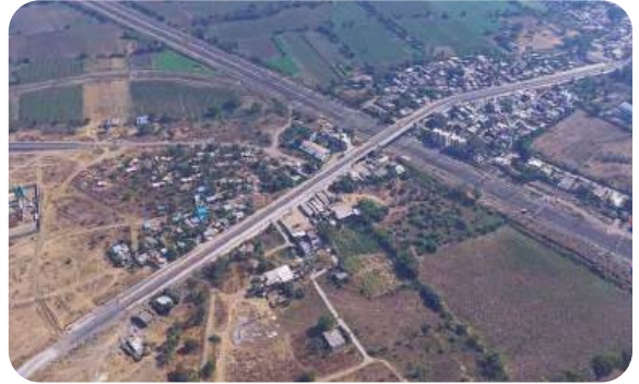
2 lane ROB at Railway Crossing (LC) – 103 Between Borkhedhi and Sindi Railway Stations in Wardha
