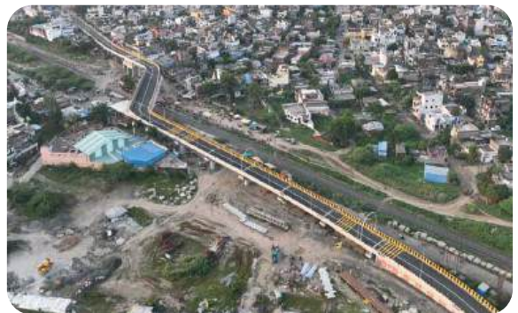
ROB at LC No. 69 between Itwari & Dighori Buzurg Railway Stations at Nagpur
