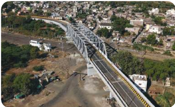
2 lane ROB at Railway Crossing (LC) – 70 Between Chandur and Dhamangaon Rly. Stations on Badnera in Amaravati
