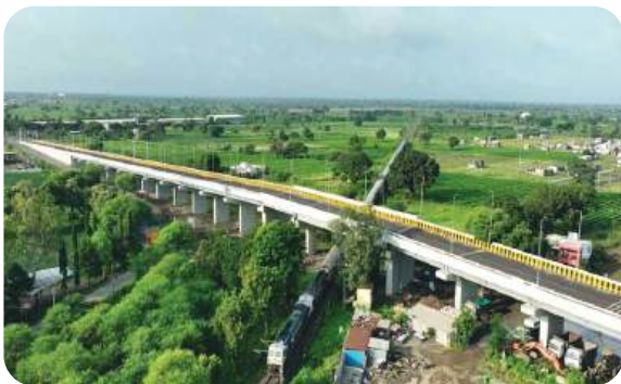
2 lane ROB at Railway Crossing (LC) – 115 Between Washim & Kekatumarg Railway Stations in Washim
