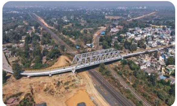
2 lane ROB at Railway Crossing (LC) – 43A/143 Between Wardha and Balharshah Railway Stations in Chandrapur
