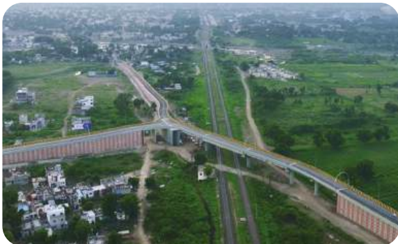
2 lane ROB at Railway Crossing (LC) – 105 Between Dondaicha and Virkhan Railway Stations in Dhule
