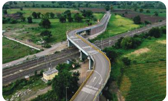
2 lane ROB at Railway Crossing (LC) – 149 Between Jalgaon & Badhali Railway Stations in Jalgaon
